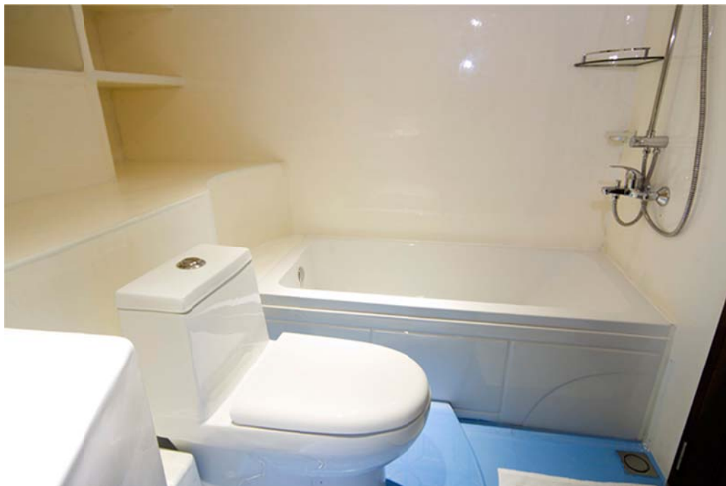
Toilet for Family Cabin
